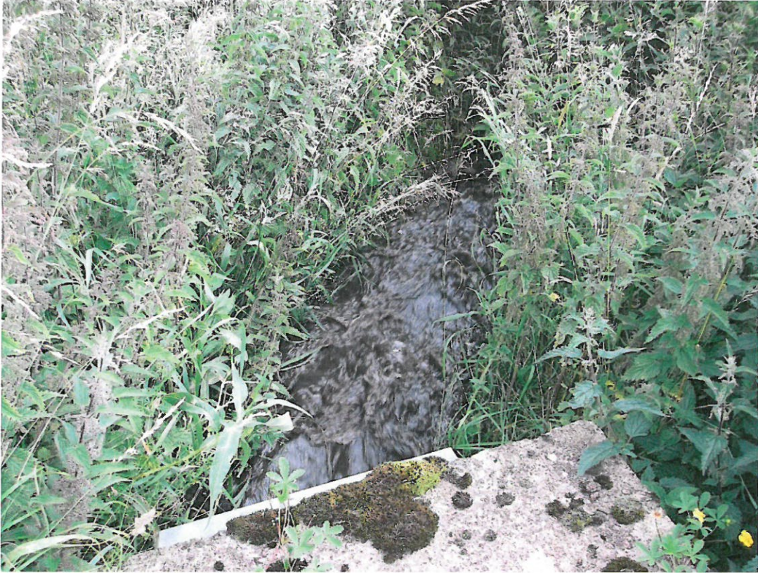
Photo11 – Outlet discharging at full capacity
