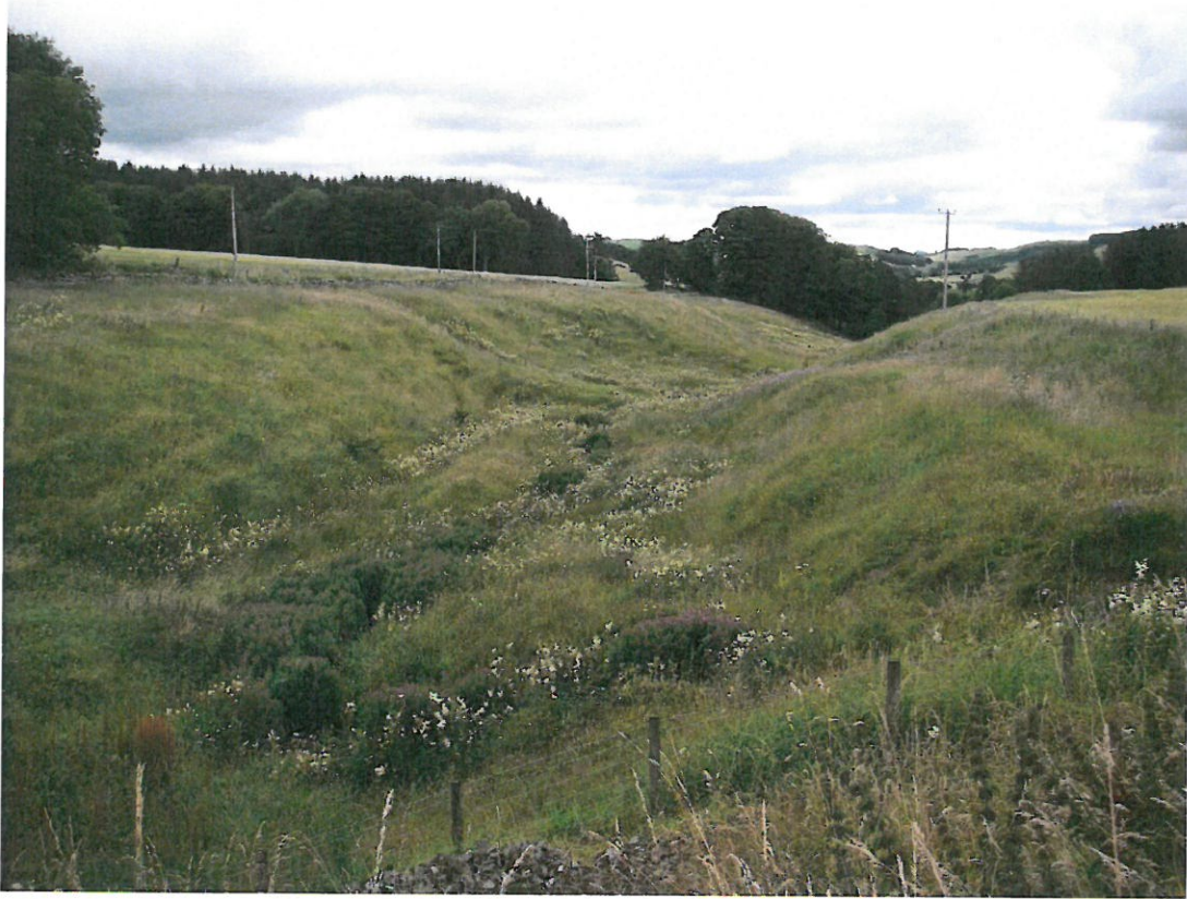
Photo 13 – Valley downstream of dam
