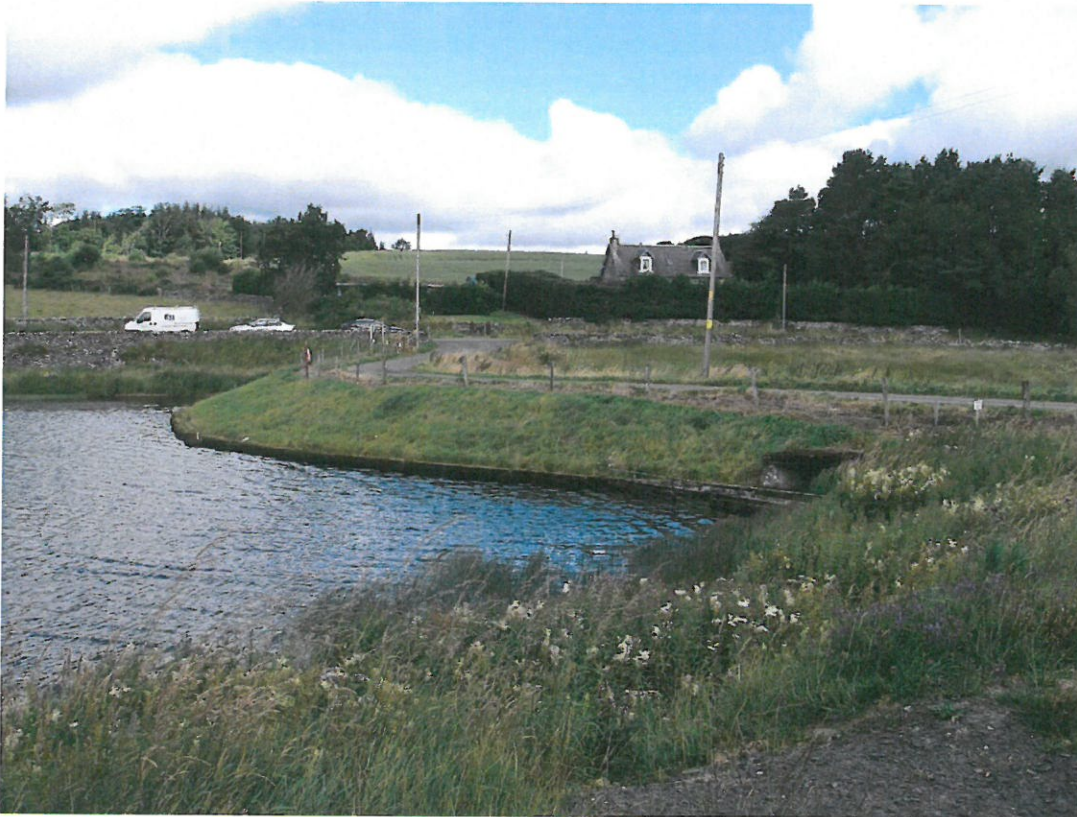
Photo 1 – Upstream face of embankment viewed from right abutment
