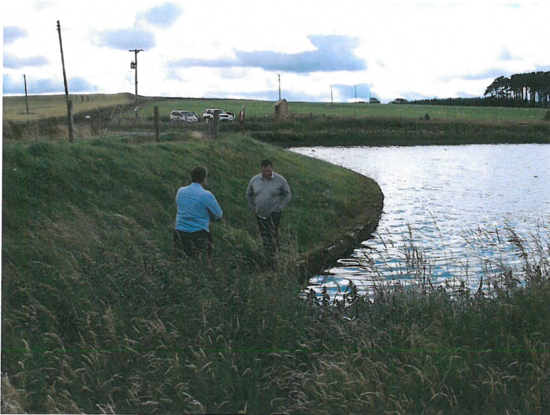
Photo 2 – Upstream face of embankment viewed from left abutment
