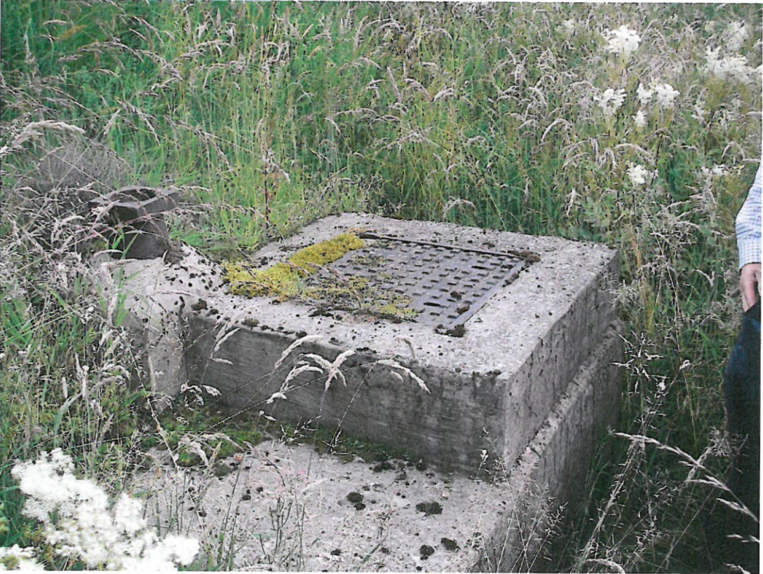
Photo 10 – Manhole on scour valve
