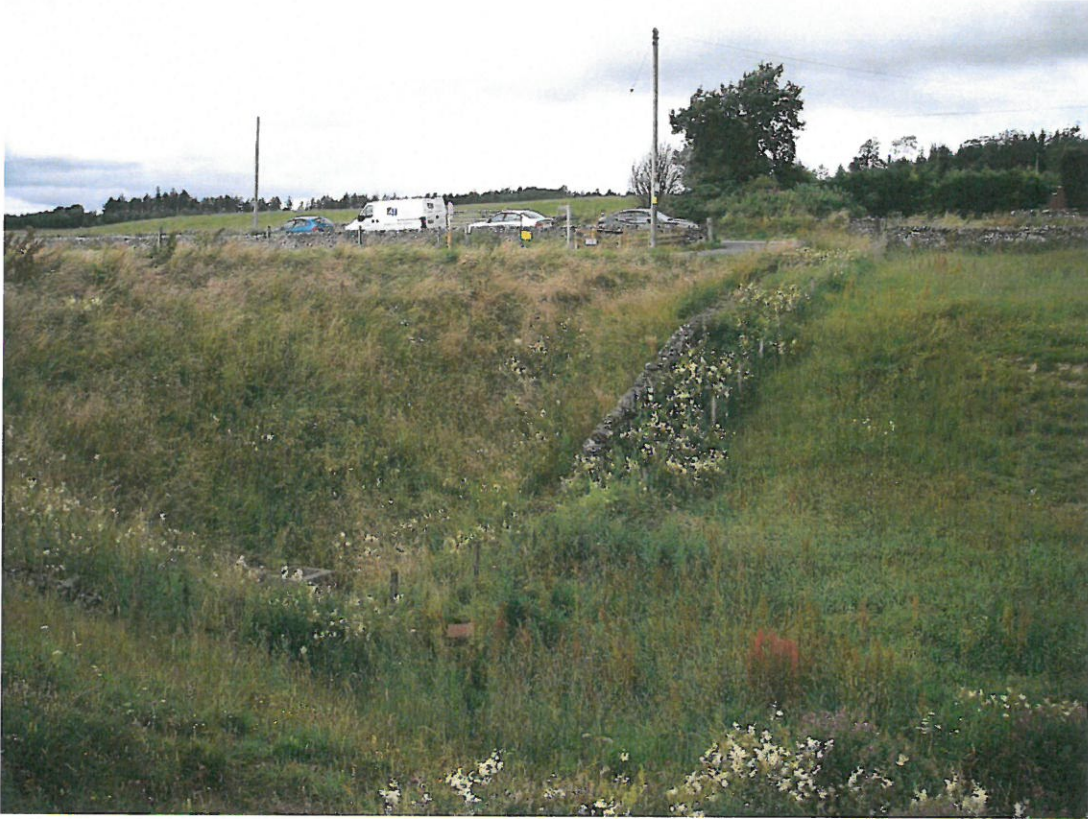
Photo 5 - Downstream face of embankment viewed from right flank
