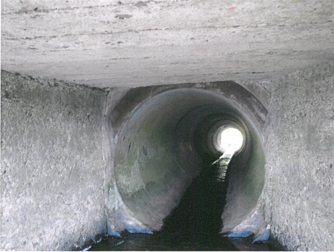
Photo 7 – Internal arrangement of 750mm dia outlet pipe (looking downstream)
