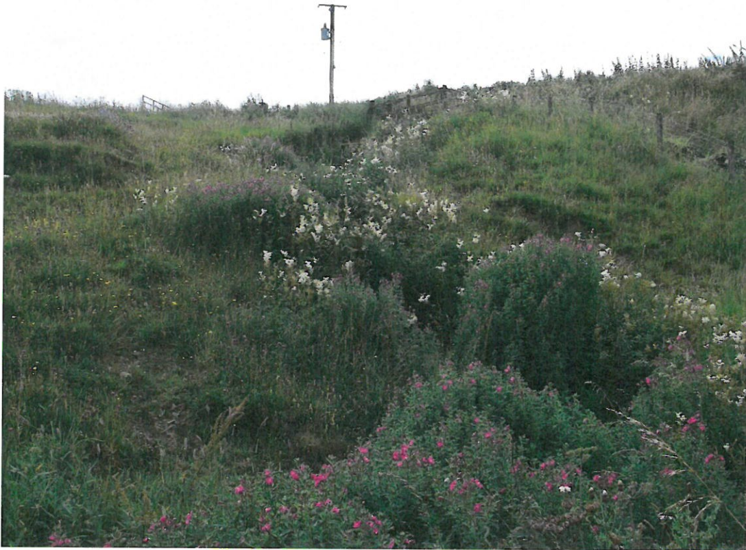
Photo 9 – Spillway channel between outlet from pipes and stream bed
