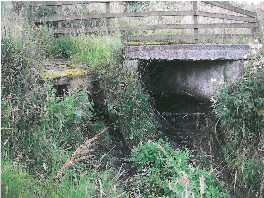
Photo 8 – Outfall from spillway pipes
